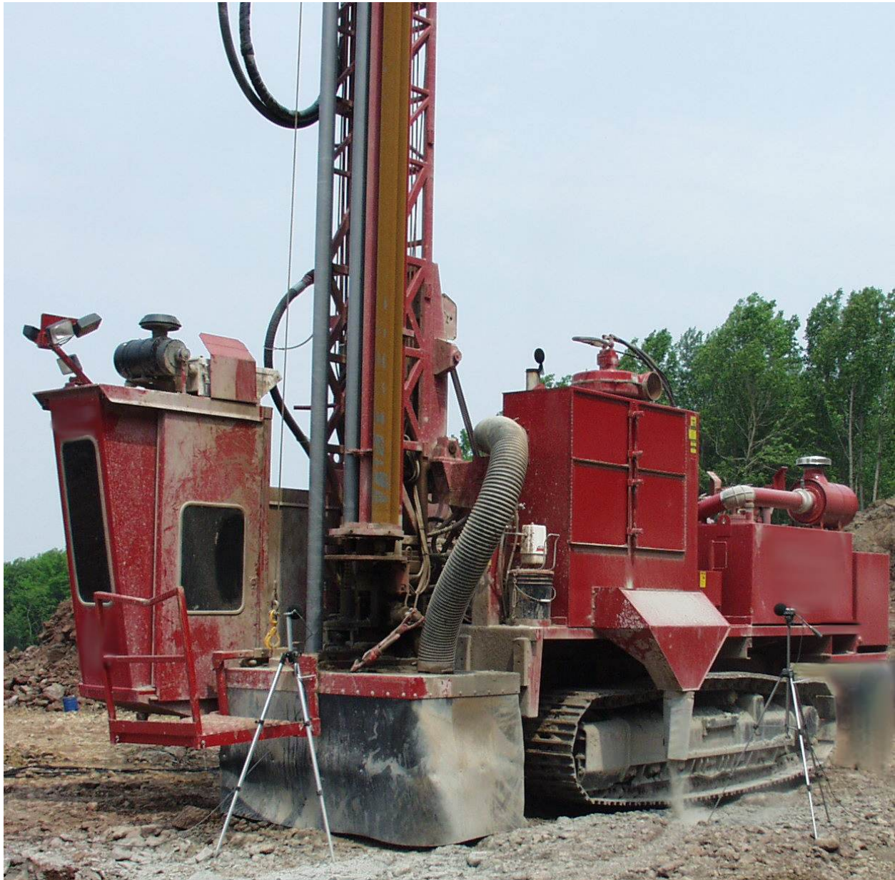
Figure 1: Track-Mounted Drill Rig with Cab.
